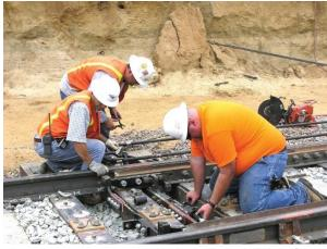
NCTD property located within the right-of-way. Specialty equipment is used to maintain the railroad right-of-way including, but not limited to, clearing vegetation away from the tracks and replacing rail ties. Track maintenance equipment and personnel are housed in a facility located in Oceanside.
